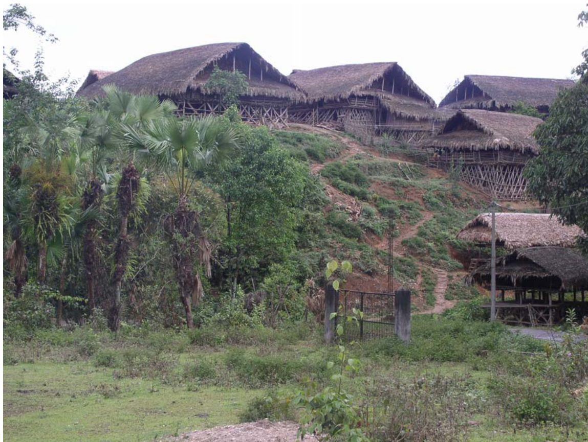
Figure 1.6 – Galo houses, with granaries in foreground (approach road to Basar town)
