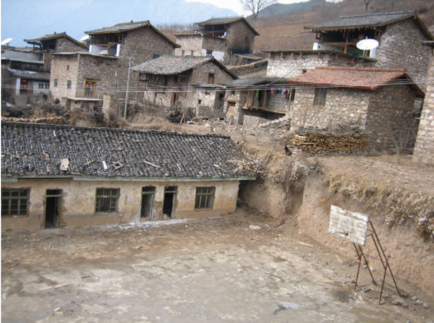
PLATE 15 A deserted primary school at Qiánxī village.
