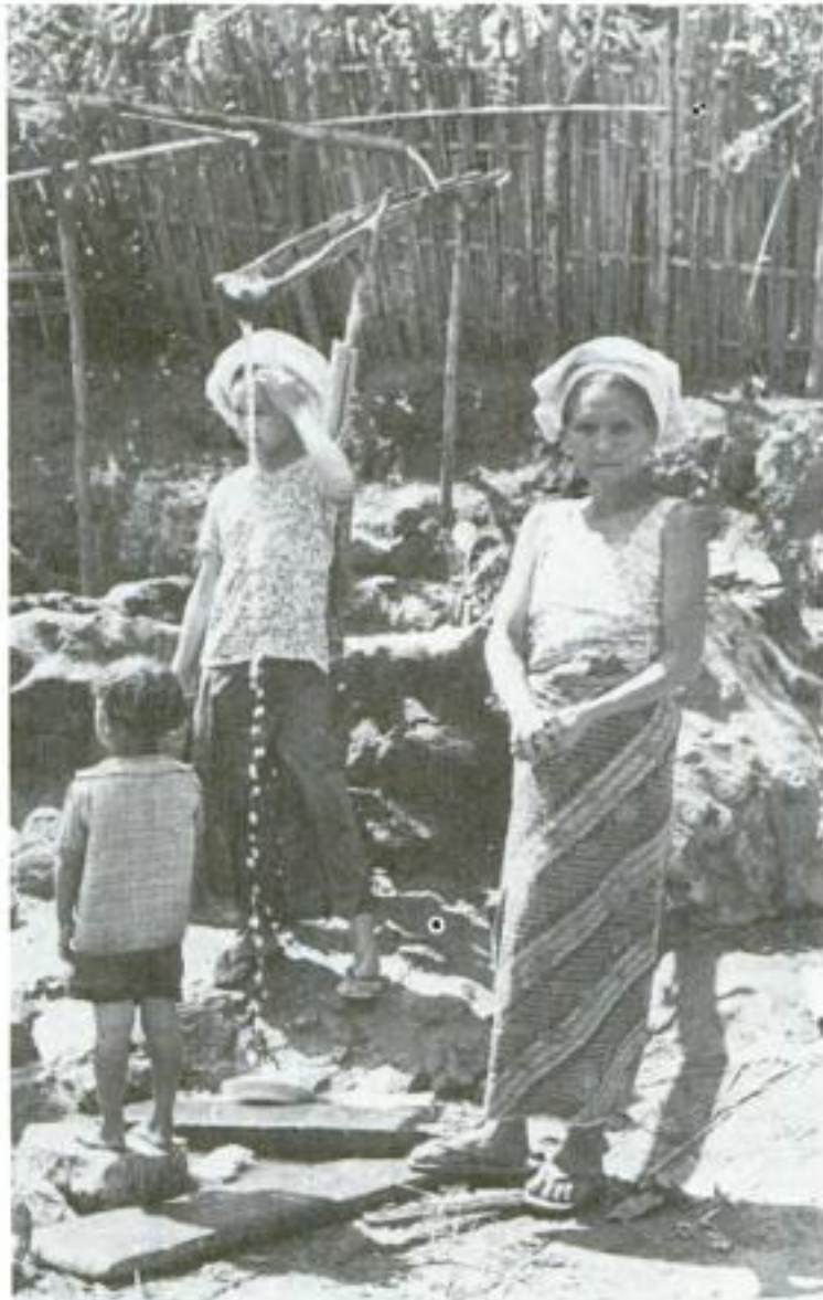
At the watering place. A system of split bamboo conduits supported by forked sticks "pipes" water for bathing and dishwashing down to the village from a stream higher up the mountain.
