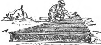
Fig. 204.—This makes a triangular mattress.
