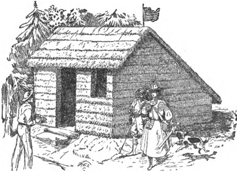
Fig. 205.—After the mats are in place the whole thing should be thatched.
