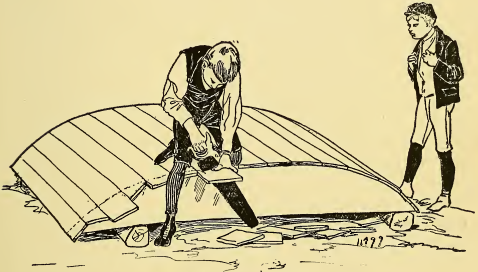
FIG. 29.—The Ends may be Sawed off Flush.
