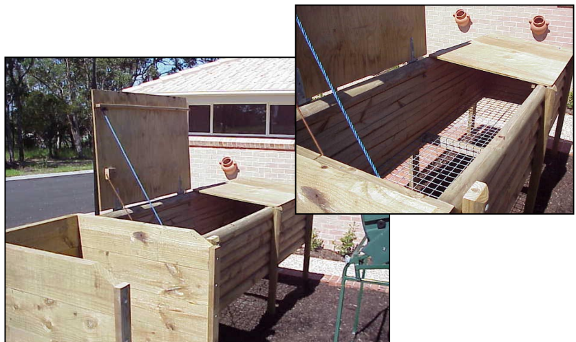
Plate 1. Example of an on-site, mid-scale vermiculture unit installation in a nursing home.
