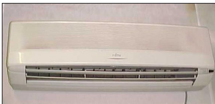
Plate 4. Example of a reverse-cycle air-conditioner used for climate control.
