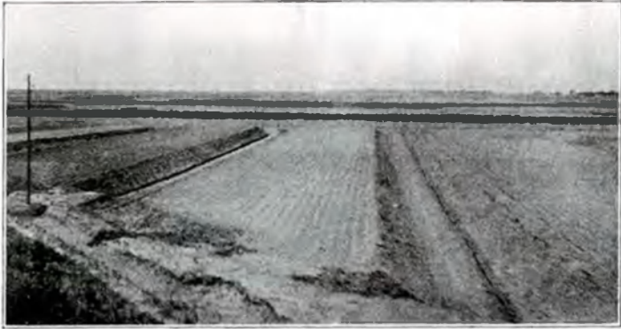
Fig. 60.—Trenching of fields for drainage, conservation of rainfall and of fertility, in the Shantung province. Trenches are two feet wide on the bottom, six or eight feet wide at the top, and two and a half to three feet deep.
