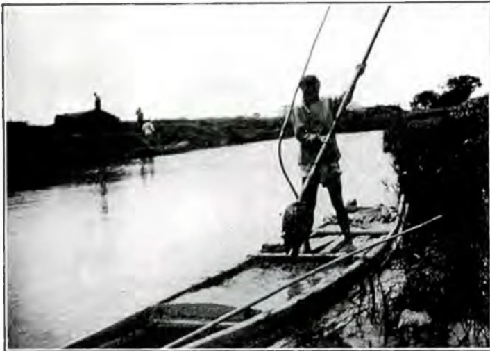
Fig. 103.—The young man is loading his boat with canal mud, using the long-handled clam-shell dredge which he can open and close at will.
