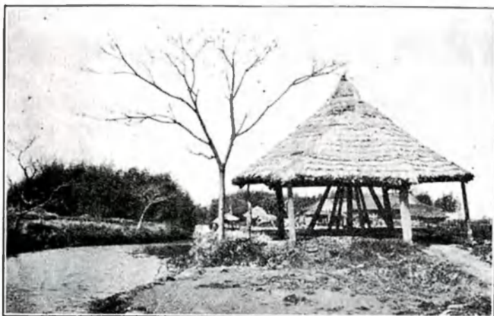
Fig. 174.—Power-wheel shelter on bank of canal, in Kiangsu province, China.
