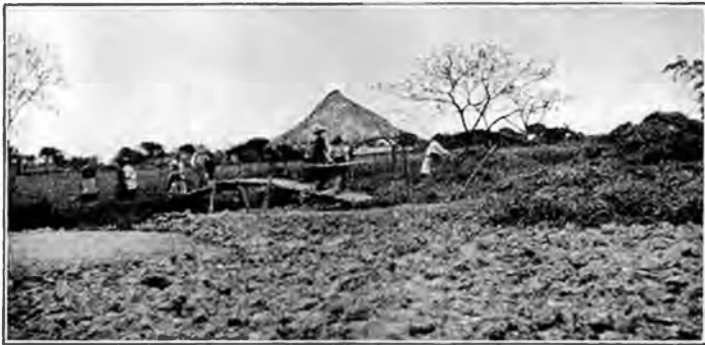
Fig. 101.—Providing for the building of a mud-and-clover compost stack.
