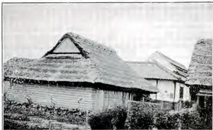
Fig. 117.—Exterior view of compost house at Nara Experiment Station.
