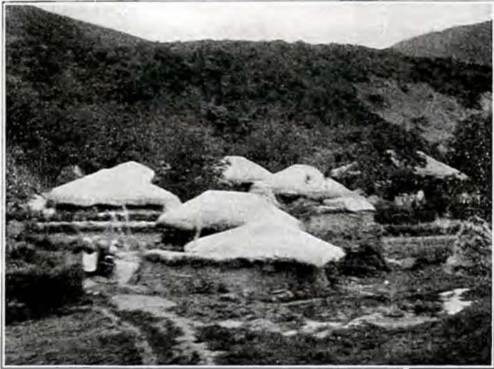
Fig. 210.—Group of Korean farm houses with thatched roofs and earthen walls, standing at the foot of wooded hills.
