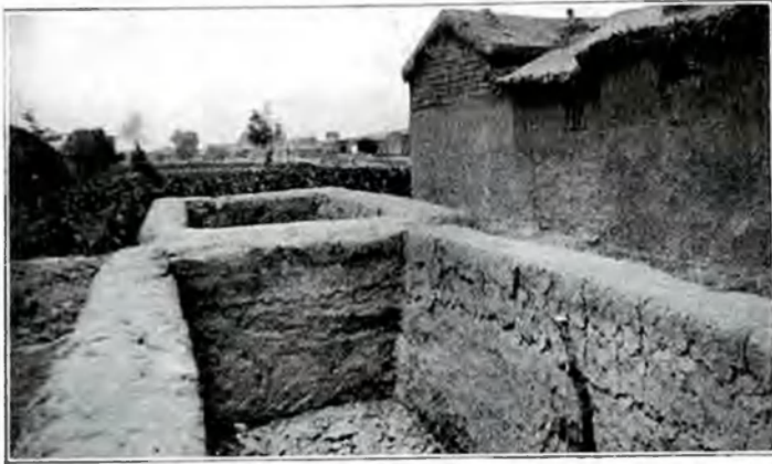
Fig. 88.—Millet-thatched roofs plastered with earth; mud chimneys; walls of houses plastered with mud, and winter storage pits for vegetables built of clay and chaff mortar.
