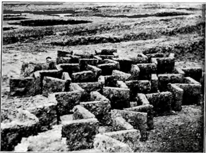
Fig. 89.—Air-dried earth brick for house building.
