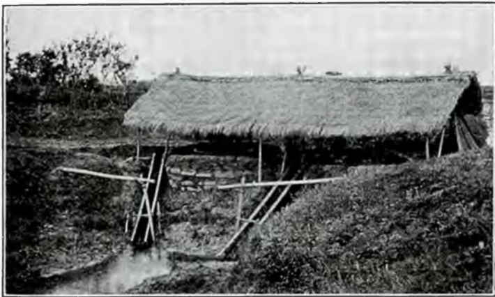
Fig. 157.—Pumping station on the farm of Mrs. Wu, showing pump shelter. two power wheels connected with pumps, set at the end of a water channel leading from a canal.
