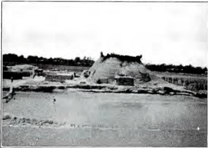
Fig. 91.—Earth and clay brick kiln on the bank of the Pei ho, using sorghum stems for fuel.
