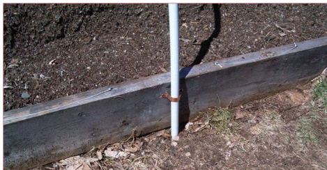
Loops on the frame of a raised bed.
