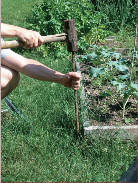
Driving the rebar into the ground.
