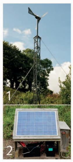
**1. Our grid-linked wind turbine** allows us to sell any excess electricity we create back to the power company. **2. Energy created** by these solar PV panels is stored in deep-cycle batteries for such things as pumping water from our spring.
