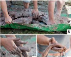
8. Keep turning and mixing the clay. 9. Test the clay to see whether it is ready to work with. Make a clay sausage. 10. Hold it with half in your palm and the other half dangling over your hand. If the clay bends but does not break, it's ready to use.
