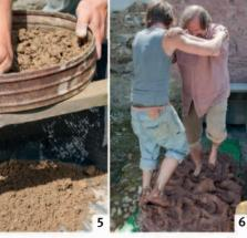
5. Sift the clay to remove pebbles and debris if you dug your clay from the ground. 6. Lay a big tarp on the ground and mix your clay—best done with bare feet. 7. Add sharp sand (about a bucketful) and some water if the clay is very dry. Mixing takes time and effort. Don't slip!
