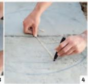
1. Build a firm base. We used some spare cinder blocks. Keep it level and build the structure up to a comfortable working height for cooking. 2. Prepare a solid floor for your oven. It must have a smooth surface. We used a couple of old paving slabs. 3. Mark the center of the oven. Make it as large as possible. Ours is about 2 ft (60 cm) in diameter. 4. Draw two circles, one 3-4 in (7-10 cm) inside the first, to show the thickness of the walls. Note the radius of the inner circle.
