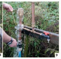
5. Attach a filter to the drive pipe to stop debris from clogging the system. Make sure it is submerged—we tie ours to a post under the water. **6. Add** an additional coarse mesh basket to stop larger debris from sticking to the filter. **7. Run** the drive pipe from the water source to the pump. 8. Connect the drive pipe to the pump. Water should flow freely through the waste valve. 9. Fix the ram pump upright. We built a frame from spare lumber and lashed the pump to it.
