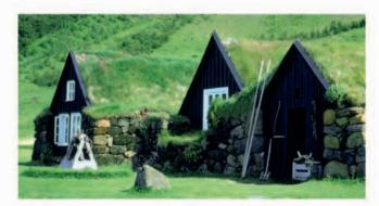
**Earth berms** can be incorporated into more familiar houses. These traditional Icelandic homes have stone foundations, timber framing, and a covering of thick sod for insulation, and can be built on level ground.
