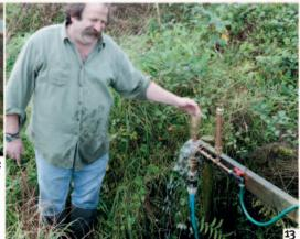
10. Unscrew the waste valve to adjust the spring. 11. Cut the spring **down** using pliers if it won't close, or add a stronger spring if it won't open. 12. Connect the delivery hose. 13. Push in the "clacker" element of the valve with a finger, to charge the ram and start normal operation.
