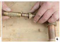
1. Make a compression joint. Slide the end nut over the end of the pipe. Slide the olive onto the end of the pipe. Push the pipe into the connector. Hand-tighten the nut onto the connector. 2. Tighten compression joints using two adjustable wrenches, twisting connector and nut in opposite directions. 3. Use the same technique to connect the pressure vessel a length of 1-in (28-mm) copper pipe sealed with the end cap. **4. Connect** the delivery check valve the same way.
