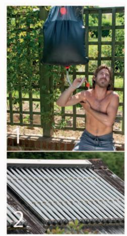
1. When we first moved to the farm, there was no plumbing, so we used a camping solar shower. This is a black plastic water carrier that is filled with water and left in full sunlight; within a couple of hours it is hot enough to provide a luxurious shower. 2. Our solar collectors comprise evacuated tubes with heat pipes connected to the manifold at the top, through which water flows and is heated.
