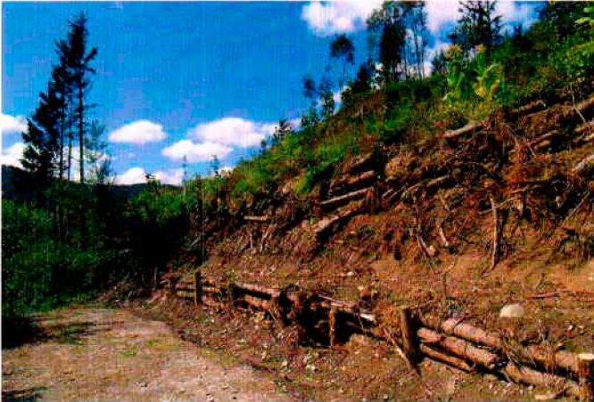
On the Krameterhof, we incorporated the fallen spruce trees into a number of structures. They were used on land that we bought from Austrian Federal Forests in 1988 which has not yet been recultivated. Shown in the photo: spruce tree trunks used to terrace and build a raised bed.
