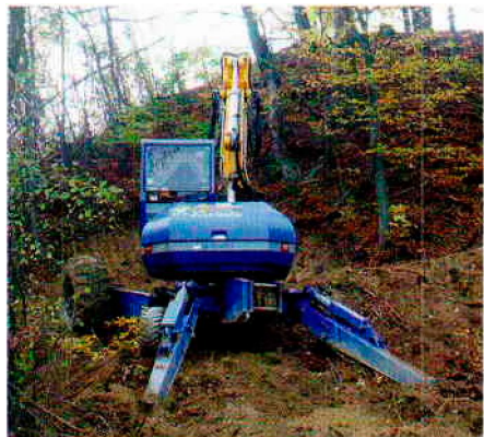
The walking excavator ('spider') can even work on rough terrain.
