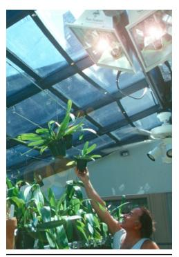
Two 1000W HPS lamps provide supplemental lighting for the hundreds of exotic orchids in this custom greenhouse. The lamps have integrated timers which turn on as the greenhouse falls into the shade cast by a nearby tree line. About a year after taking this photo, the author paid another visit and found two more lamps installed and nearly double the number of plants. I guess gardening kind of grows on you!
