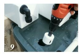
**Step 9.** Using a 1.5" hole saw, cut a hole for each chamber's drain fitting to mate with the lid of your reservoir. I have found the simplest way to measure and mark off the location for these holes is
