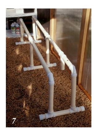
**Step 8.** Now that your stand is complete, you can put the Dutch Buckets into place by fitting the drain nipples into each of the 1" holes in the drain rail.
