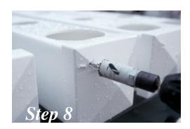
**Step 8.** Using a 1 3/8" hole saw, cut a hole into each of the endcaps to accommodate the spray lines. Center this hole exactly 1 1/8" down and 1 1/8" over from the same corner the spray line clips are attached. You will use a 1" I.D. rubber grommet (shown in the next step) to seal the compression fitting as it passes through this hole.
