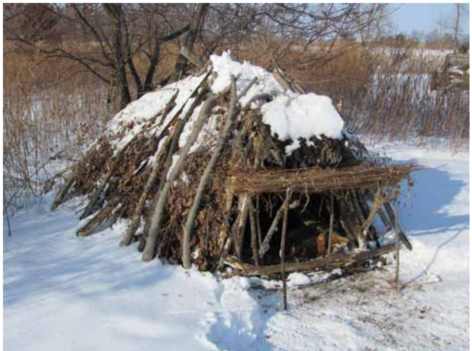
Side view of branches holding debris in place.
