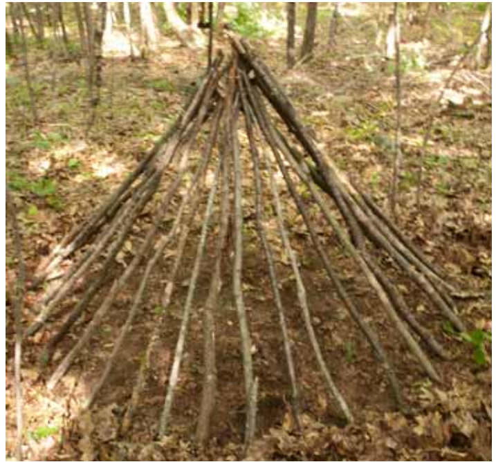
Lean ribs on the tripod making its circle footprint.
