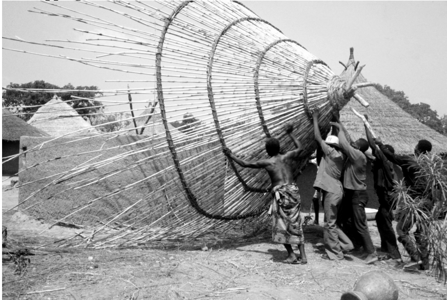
Photo 1. Tipping a roof in Askaen
