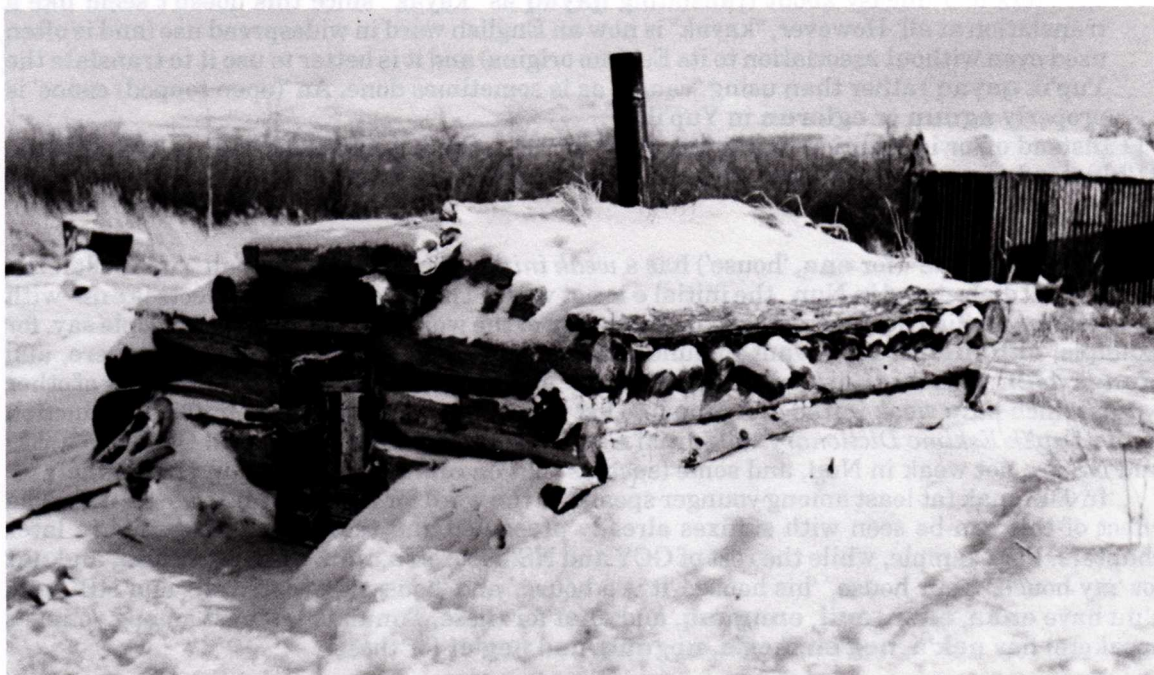
Steambath house, maqivik , in Marshall, 1968. Water is poured on heated rocks to make steam. In older times, dry heat was produced by building a fire in the communal men's house, qasgiq . With the abandonment of the men's houses in most areas, the word qasgiq has become synonymous with maqivik . Photo by Steven A. Jacobson.
