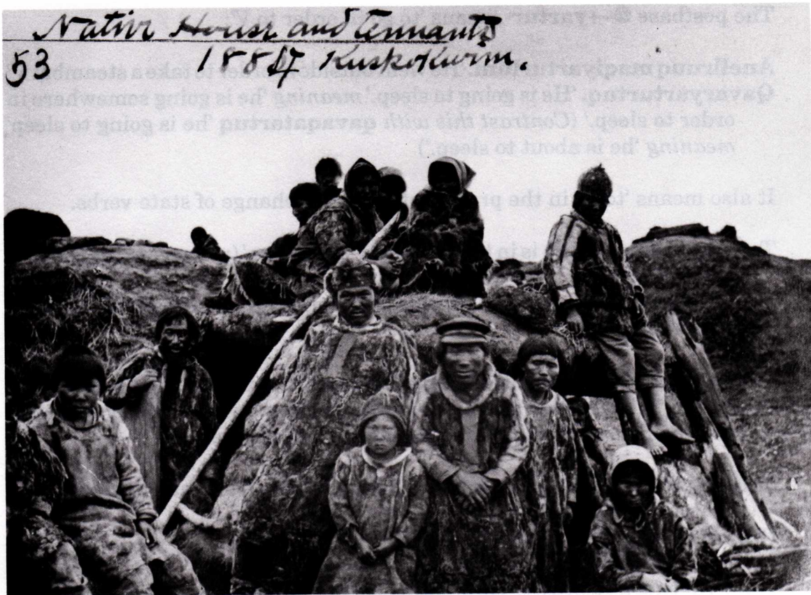
Semi-subterranean sod houses were well insulated and could be built from local materials even in treeless areas, but were subject to spring flooding. Joseph H. Romig Collection (acc. #90-043-881) in the Archives, Alaska and Polar Regions Dept. UAF.
