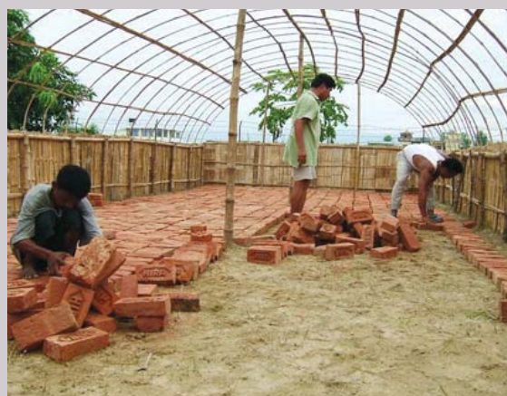
Figure 5. Floor work for growing house
