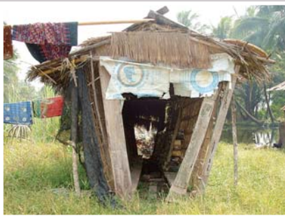
Figure 24. Imperata grass roof with two stacks of substrate bags as the walls
