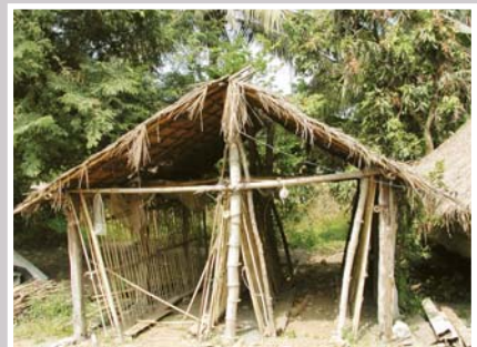
Figure 32. Rack frame structure
