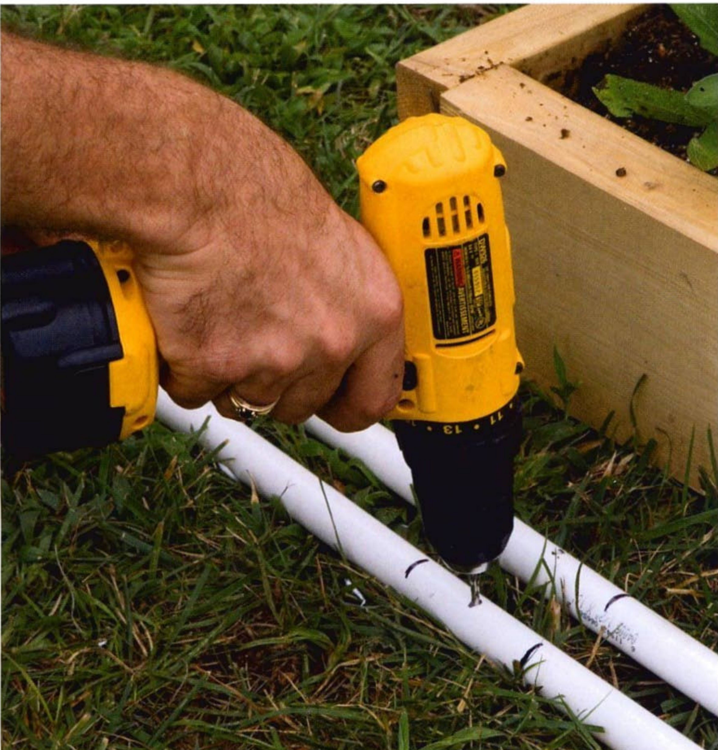
Drill one hole in the center of two 10-foot PVC pipes.
