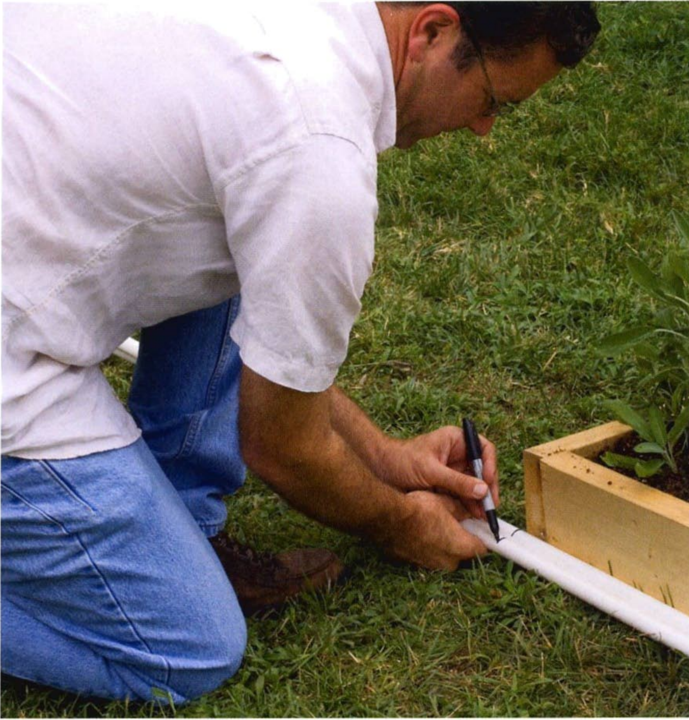
Locate the center of your two ten foot pipes.
