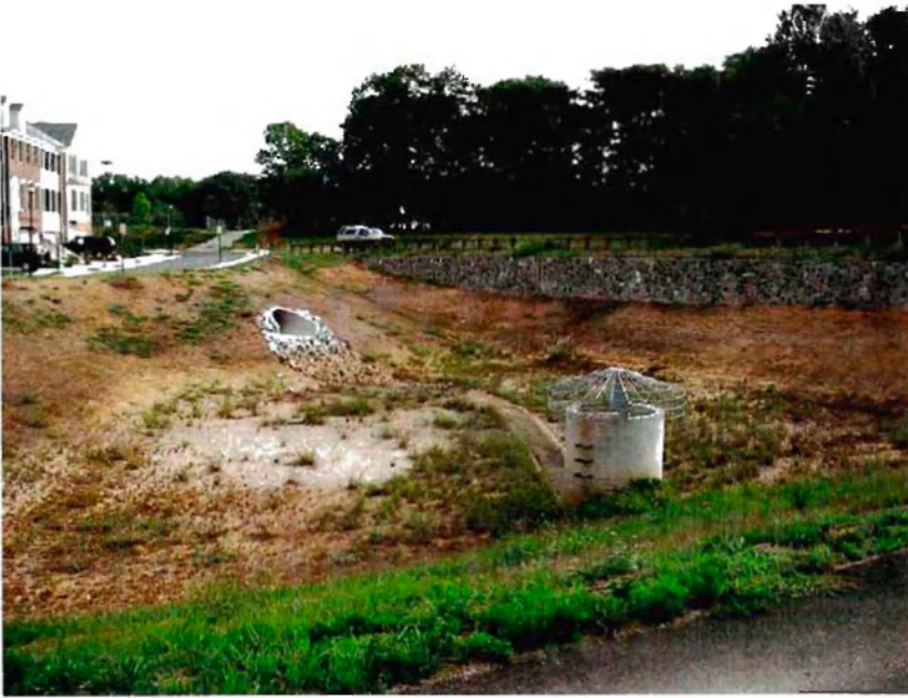
Figure 6.34 A standard retention pond such as is built in most new developments to comply with the stormwater regulation. It requires huge investment, and needs to be maintained properly.
