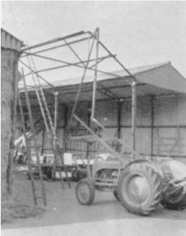
Building construction with the aid of a tractor
