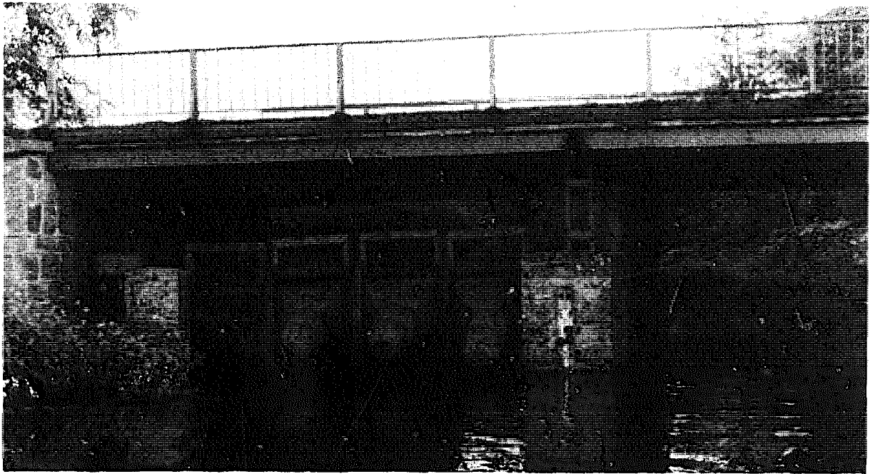
Fig 254 Permanent barrier in the river Eider in northern Germany at the outlet of a lake (Westensee), with baskets made of iron.
