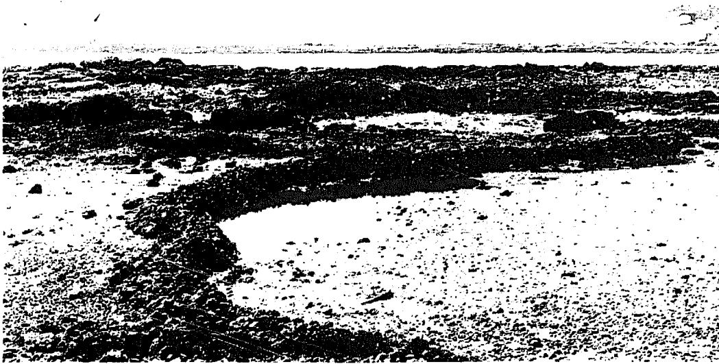
Fig 256 Stone dam built off the coast of Guinea to capture fish as the tide falls.
