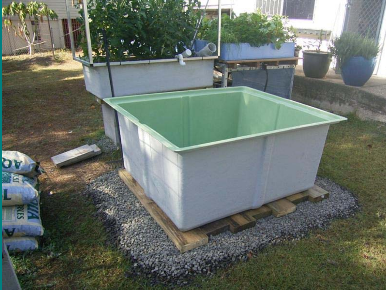
The tank is positioned on the platform.
