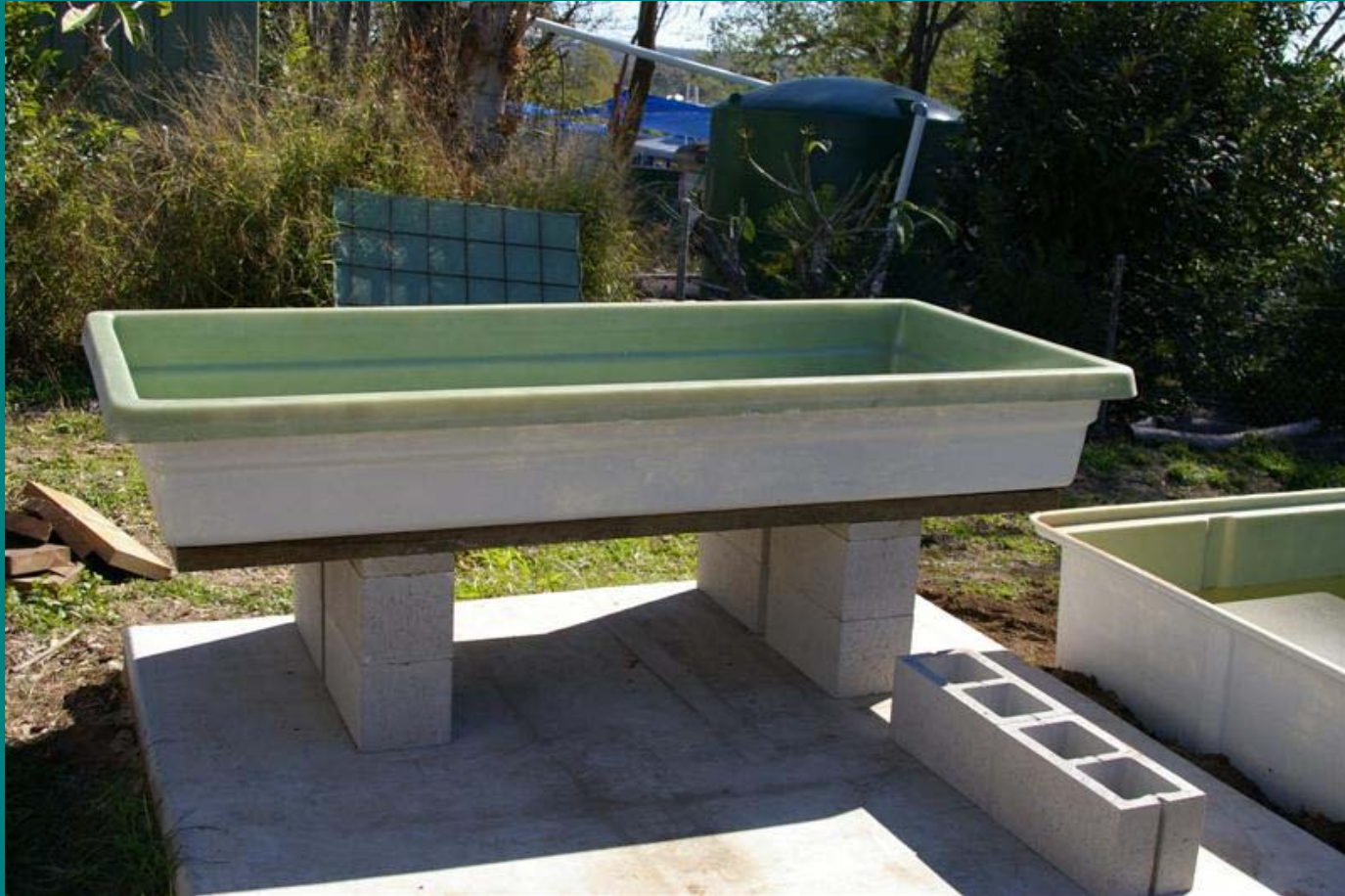
The first 500 litre fibreglass grow bed in place.
