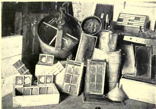
Extracting-room showing extractor, strainer, uncapping can, bee-escape, smoker, uncapping knife, gloves, funnel, supers and sections, extractor pocket containing extracted sections, partly filled sections as yet uncapped, extracting frame with comb, etc.
