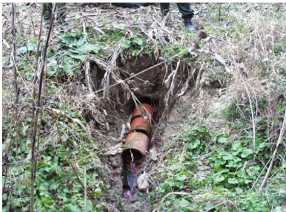
Land application on fields with sub-surface drainage tiles could result in a discharge.
