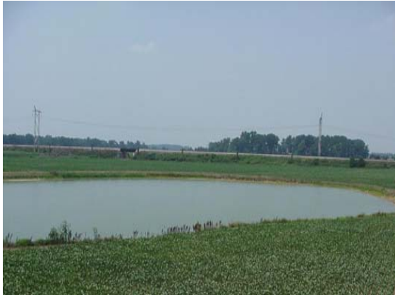
Well designed and maintained layer wastewater lagoon.
