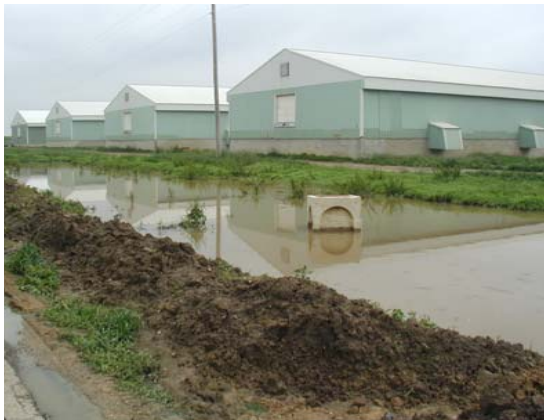
Poorly maintained facility affects storm water management.
