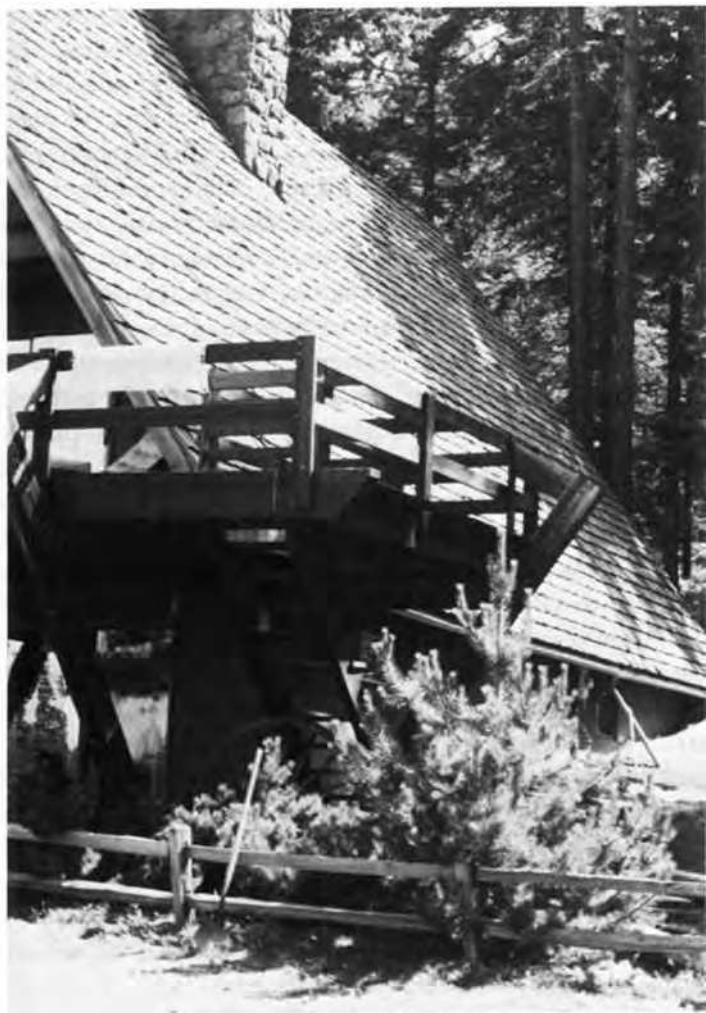
This home also serves as a survivalist's retreat. It was built with twelve-inch concrete walls in the basement and butted into the side of a hill. Trees provide camouflage and fuel for cooking and heating via the fireplace.
