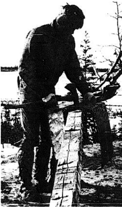
Figure 13.10 - Forming the stove body on a squared iog.
