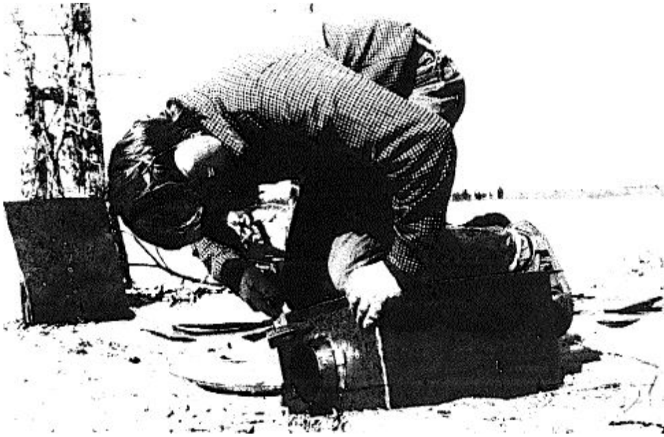
Figure 13.17 - Mounting the stove bottom.
