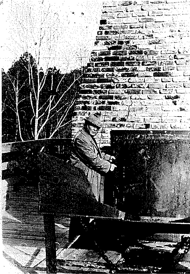
PLATE 20 Professor Ray Farabee indicates the charging point of the old Tannehill furnace. Professor Farabee was the furnace master for the refiring of the old furnace.
