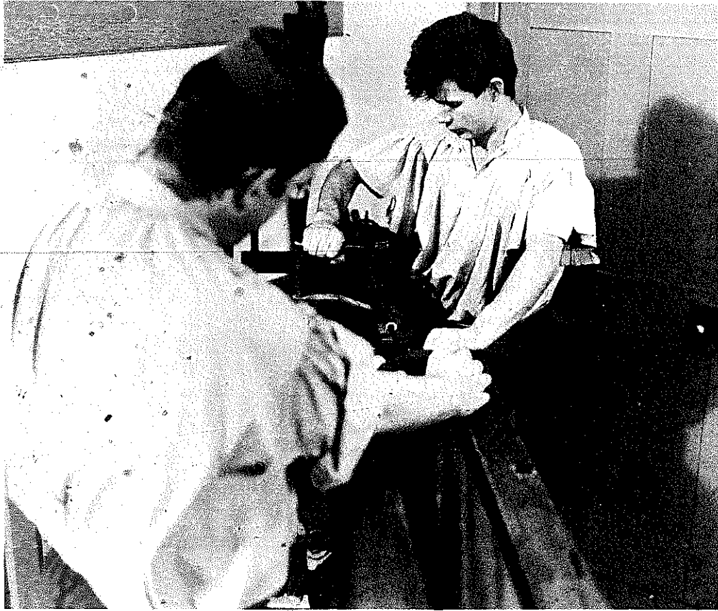
PLATE 184 Wallace Gusler and his assistant preparing to rifle a barrel. (Photo courtesy of Colonial Williamsburg.)
