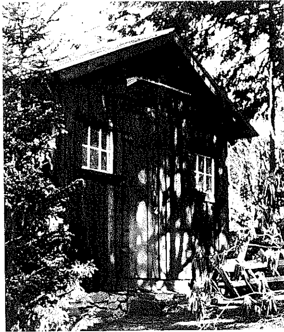
PLATE 324 The front of Joe's shop.
