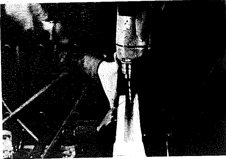
PLATE 259 Hershel drills feeler holes to make sure that the long drill bit drilling the ramrod hole is on course.
