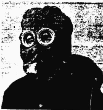
FIG. 110.—British Hypo, P., or P.H. Helmet in use, skirt buttoned under tunic.
