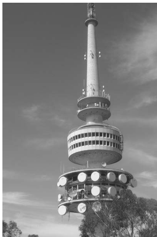
Figure 10.1c Central trunking site (Black Mountain, Canberra, Australia).
