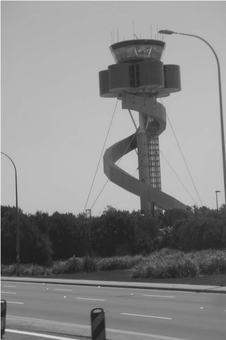
Figure 10.26 Example control tower with VHF antennas on the roof.
