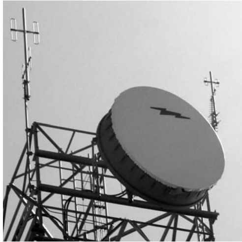
Figure 10.24 High performance parabolic antenna (see Shrouds). Reproduced from Gabriel Electronics.
